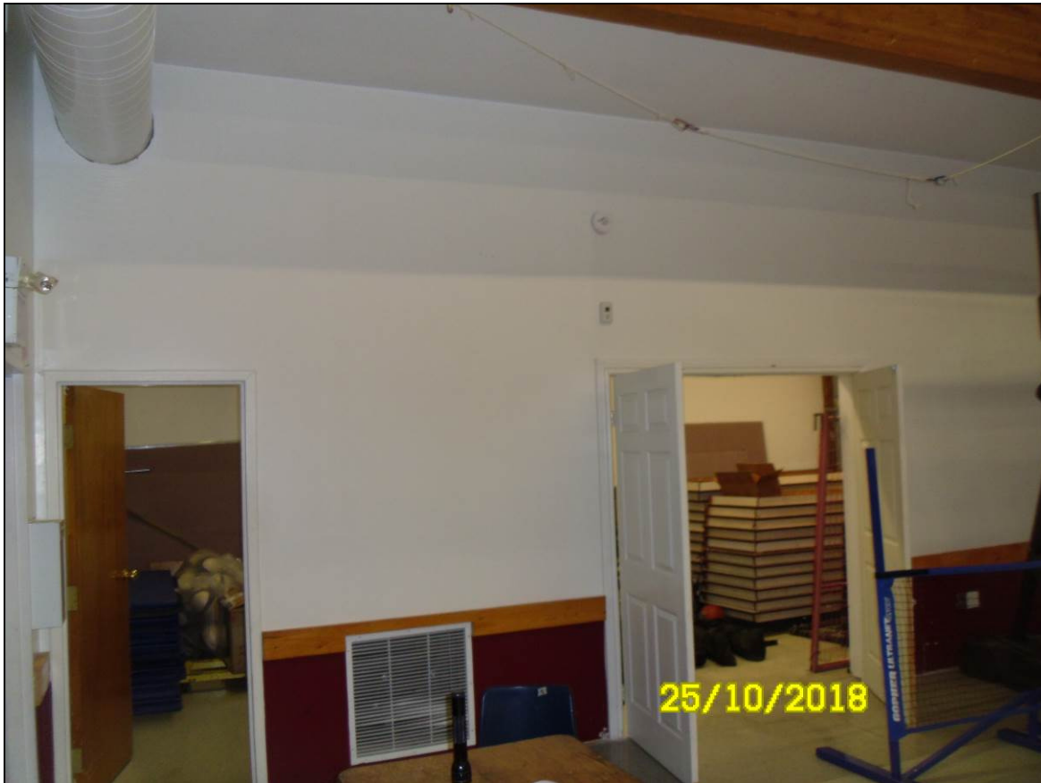
Photograph 1: View of drywall walls with asbestos-containing drywall joint compound in the Auditorium (Location 5). Off-white wall paint throughout the second floor of the building was found to contain <0.1% by weight and is considered a low-level lead paint.
