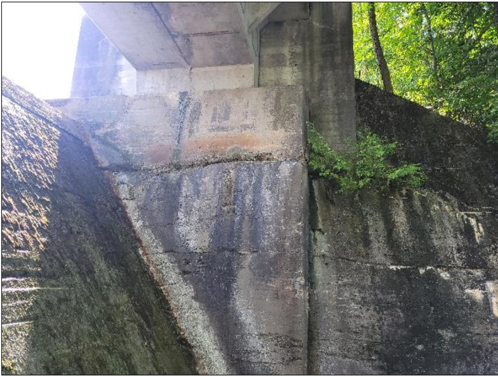
Abutment and south wingwall; Delamination at cold joint.
