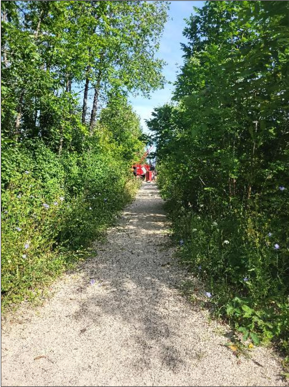
Crest, looking north. Vegetation on both upstream and downstream embankments.
