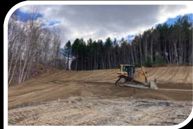
Slopes stabilization (October 2022)
